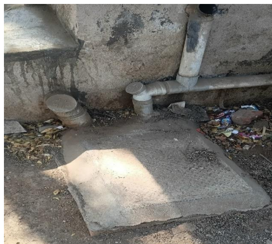
Septic tank near toilet of main building
