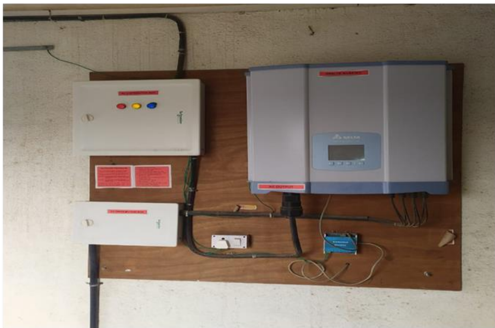
Solar on Grid Invertor
