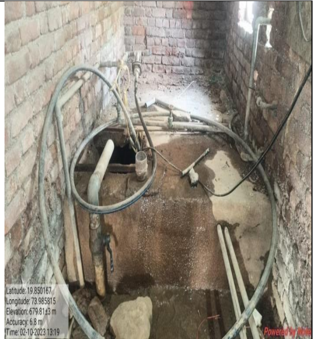
Water Storage Tank
