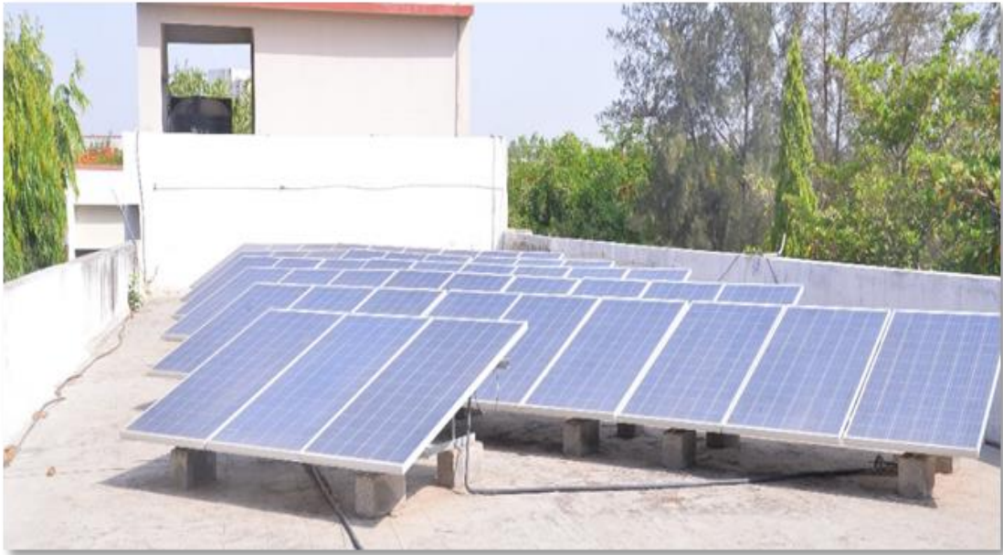
Top Solar Off Grid Solar System (7.5 kWh)
