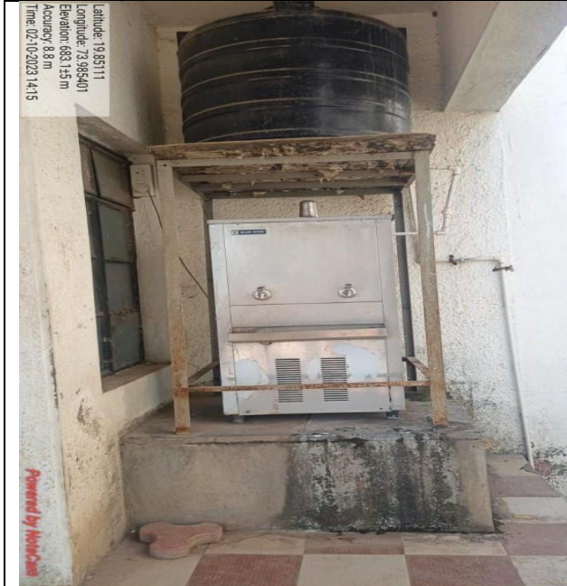
Water Storage Tank
