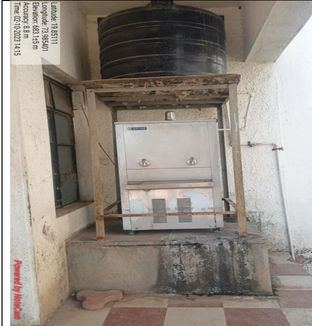
Water Storage Tank
