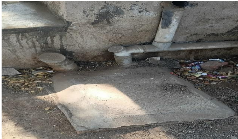
Septic tank near toilet of main building
