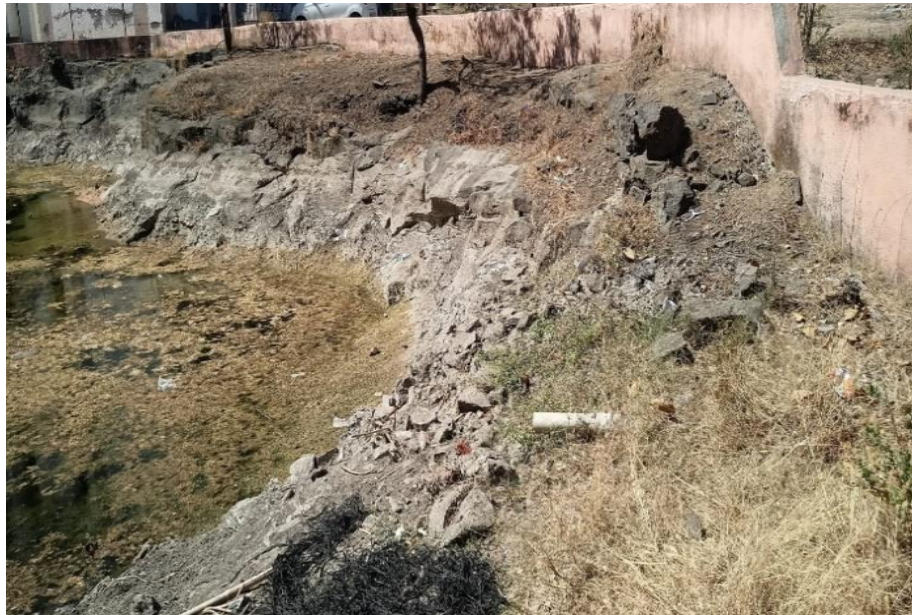
Rain Water Harvesting Installation unit (Work in progress)
