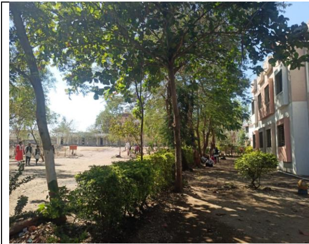
Back Side of the Main Building
